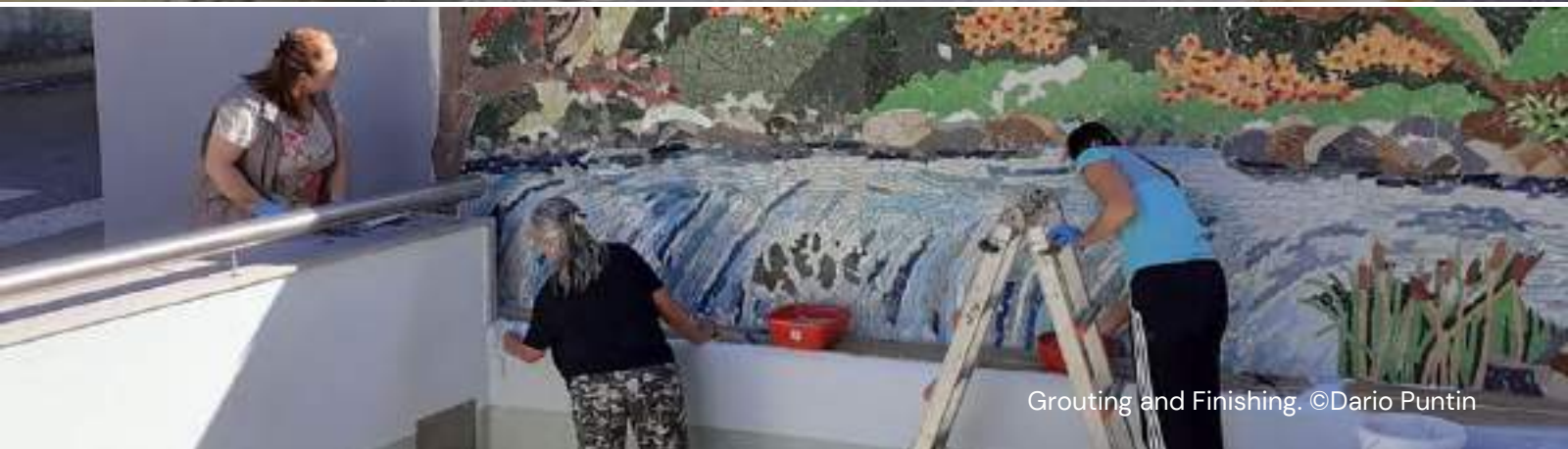
Grouting and Finishing. ©Dario Puntin
